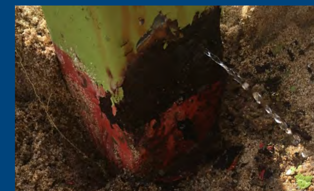
Play equipment (rusted post) at Ken Cantwell
