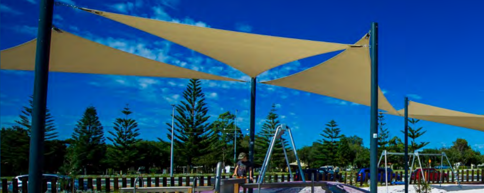
• Shade sails over Koombana Foreshore Playground
