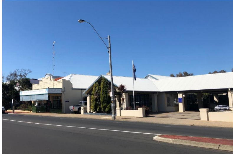
Figure 4 is a recent photo showing the reconfigured front elevation with the garage door removed and new glazing installed. Also indicated is the funeral chapel and porte cochere constructed circa 1990.
