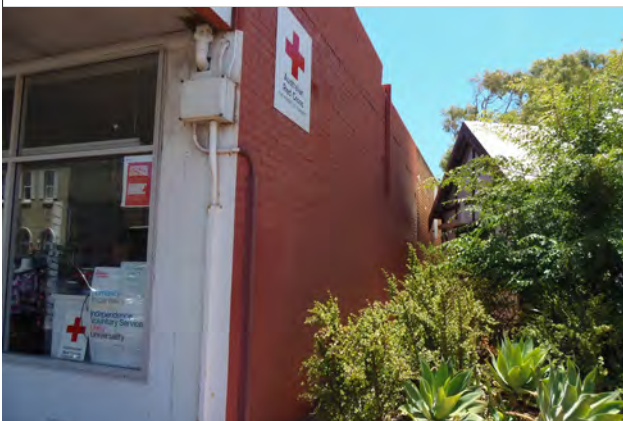
Eastern facade. Source: SCA 2022
