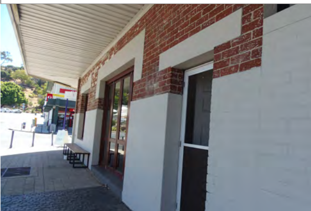
Corner exposed brickwork. Source: SCA 2022
