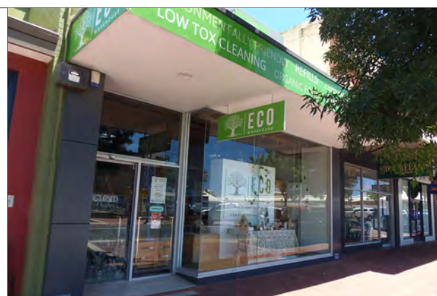
Shop front. Source: SCA 2022
