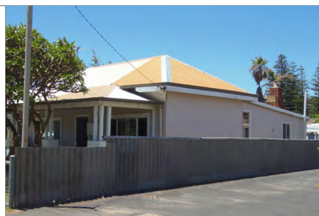
Western facade. Source: SCA 2022
