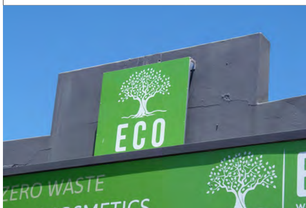
Parapet. Source: SCA 2022
