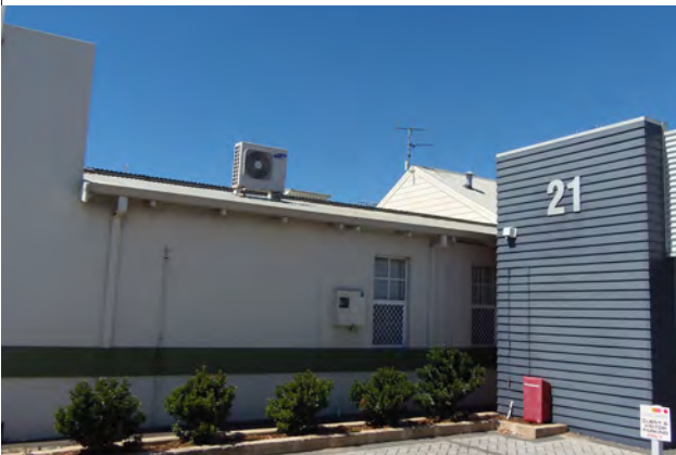
Southern facade (original building to the rear). Source: SCA 2022
