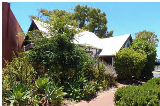
54 Wellington Street. Source: SCA 2022
