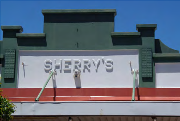
Parapet. Source: SCA 2022
