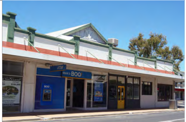
Victoria Street facade. Source: SCA 2022
