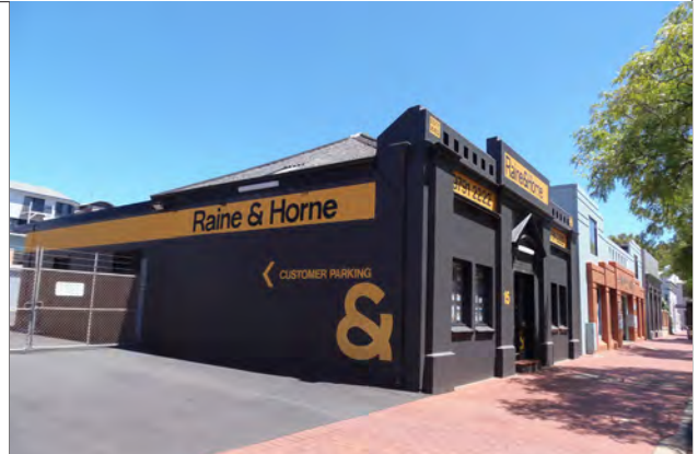
Southern facade. Source: SCA 2022
