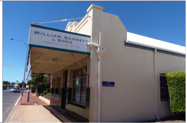
Northern Building's south facade and parapet. Source: SCA 2022
