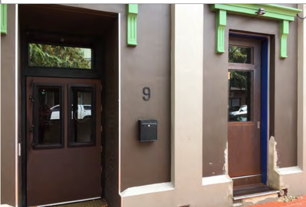
New door addition. Source: City of Bunbury June 2022
