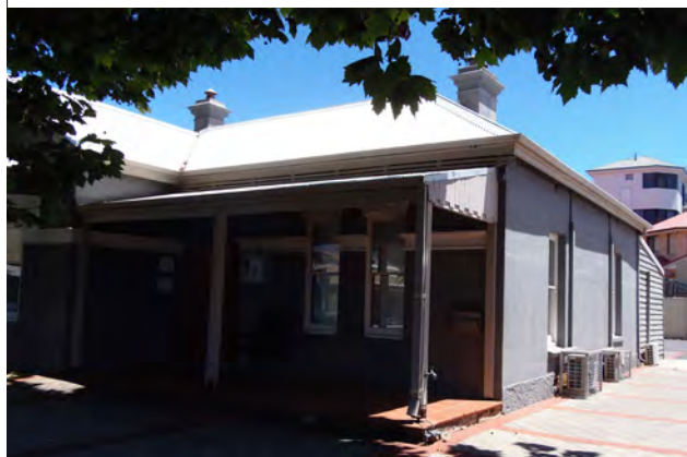
Front verandah. Source: SCA 2022
