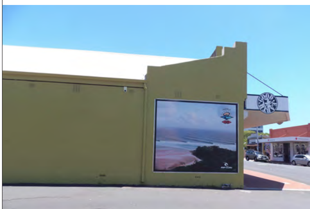
Eastern facade. Source: SCA 2022
