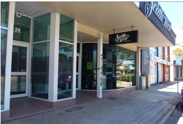
Shop front. Source: SCA 2022
