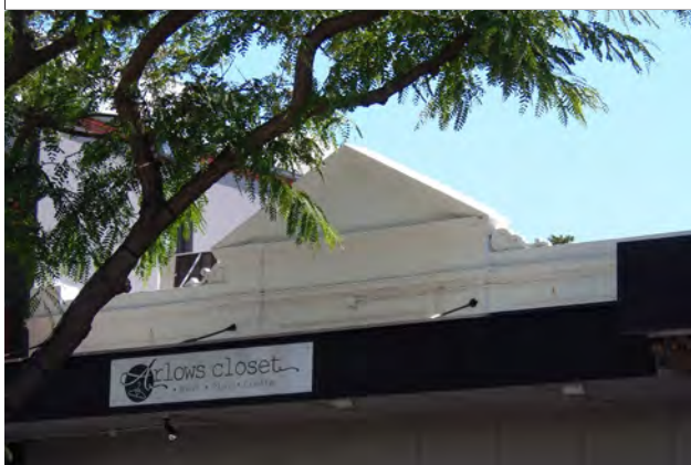
Parapet. Source: SCA 2022
