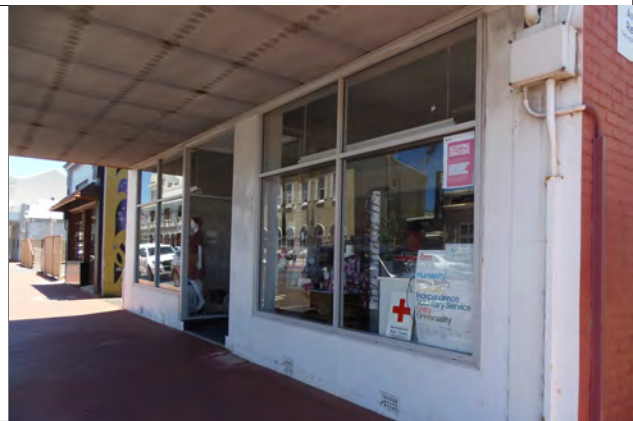
Shop front. Source: SCA 2022
