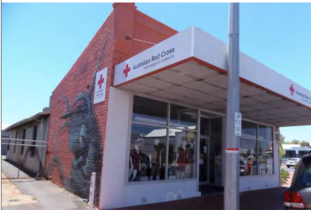
Front facade. Source: SCA 2022
