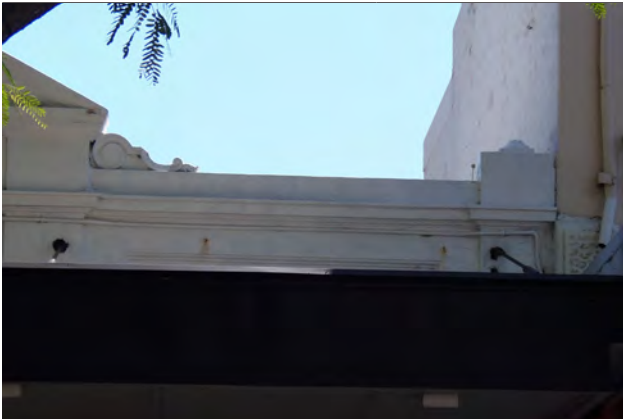
Parapet connection to neighbouring Lyric theatre. Source: SCA 2022
