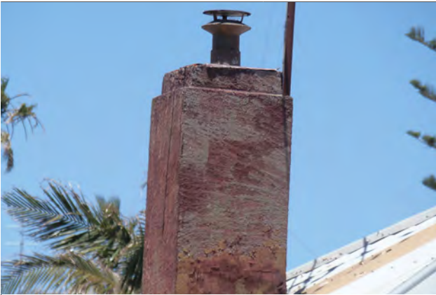
Chimney. Source: SCA 2022
