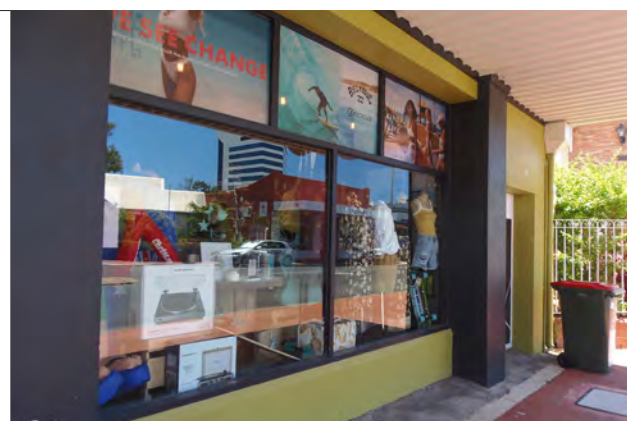
Shop front. Source: SCA 2022
