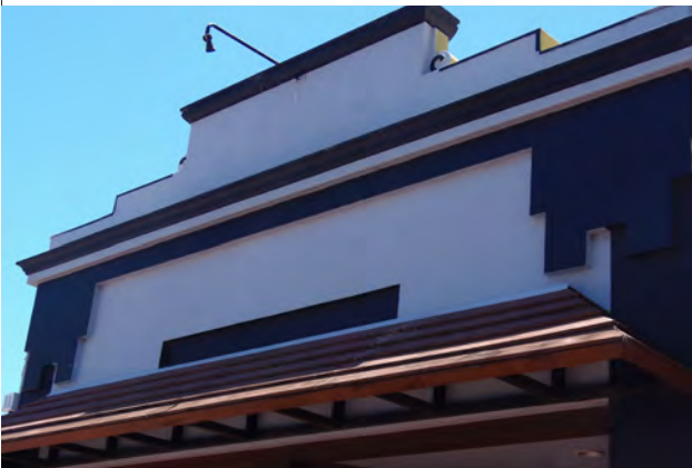
Parapet. Source: SCA 2022
