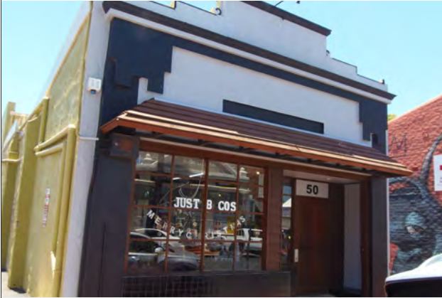
Front facade. Source: SCA 2022
