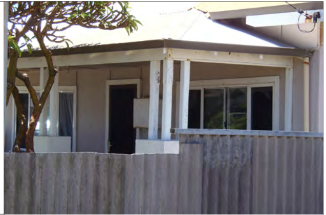
Front verandah. Source: SCA 2022
