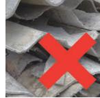
Asbestos and fence panels
