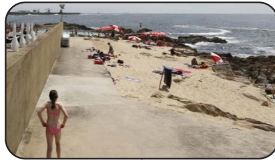
Protected walk & Building Plinth
