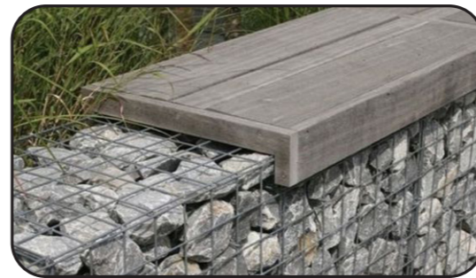
Repurposed basalt in gabion wall over quarry wall
