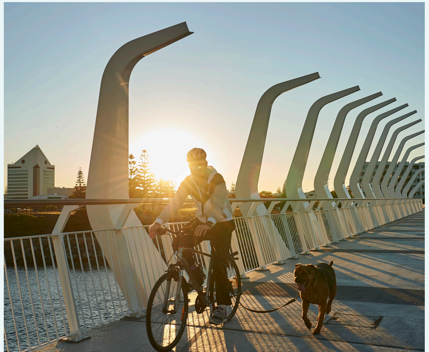
Koombana footbridge, Regional Park, Bunbury
