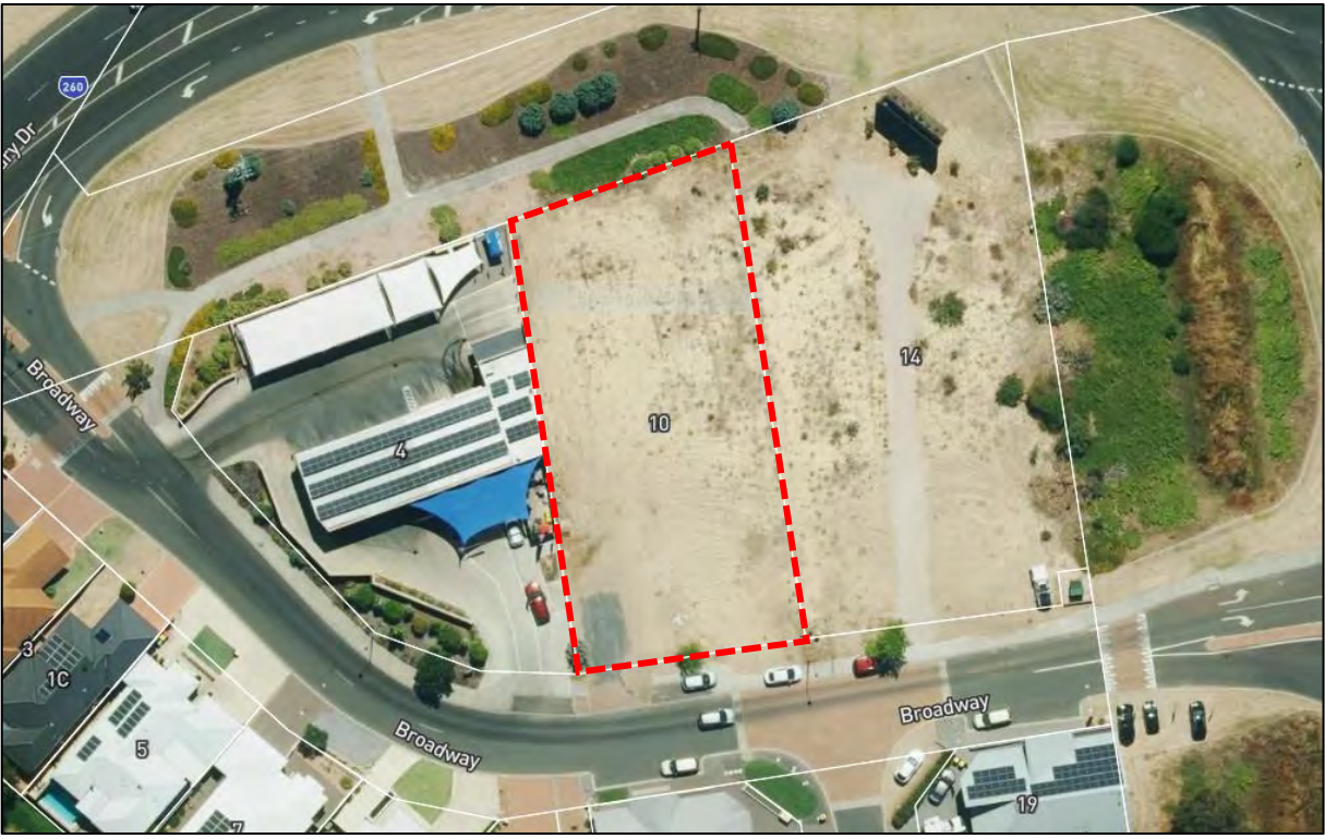
Figure 2: Aerial View (March 2022)
