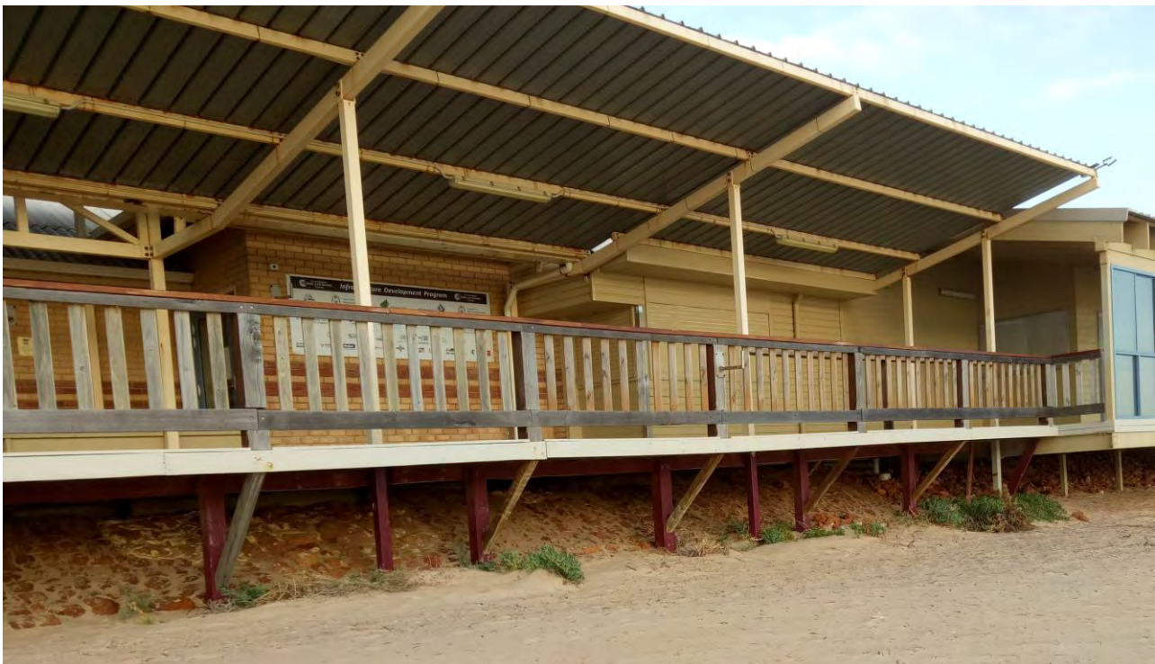
Figure 5-1 Revetment beneath Bunbury Surf Life Saving Club, June 2021.
