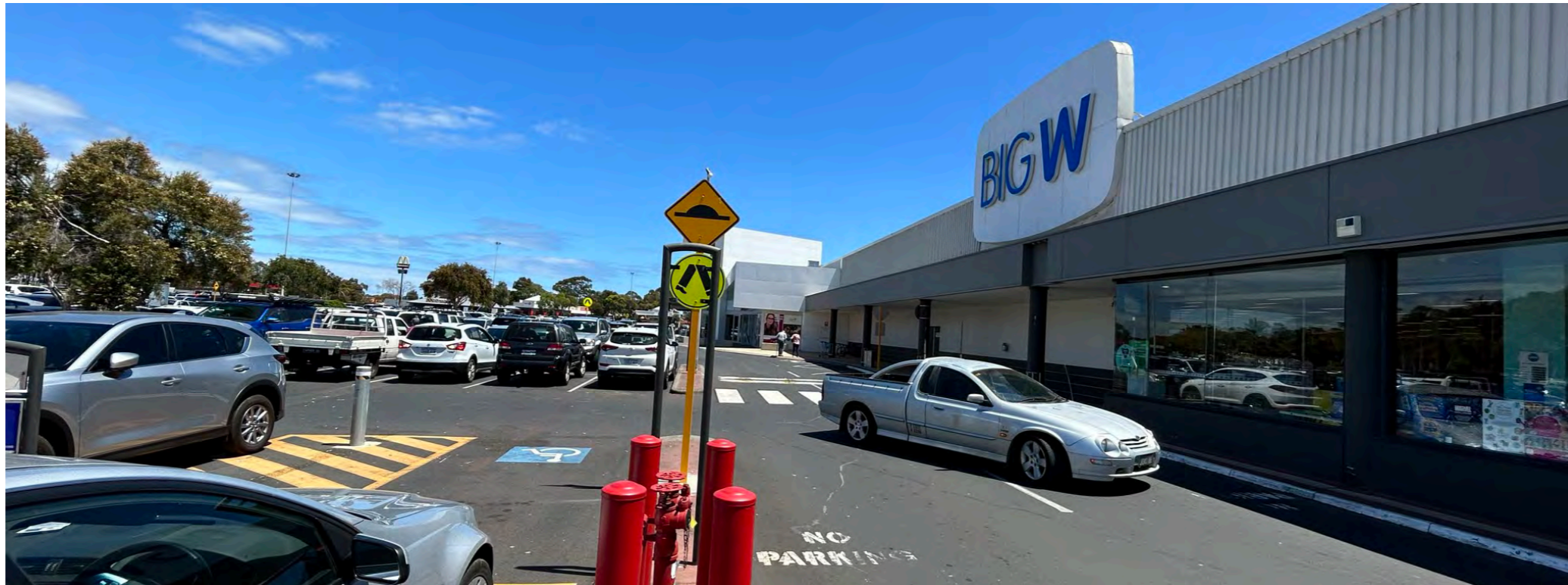
Southern Elevation - Big W Facade
