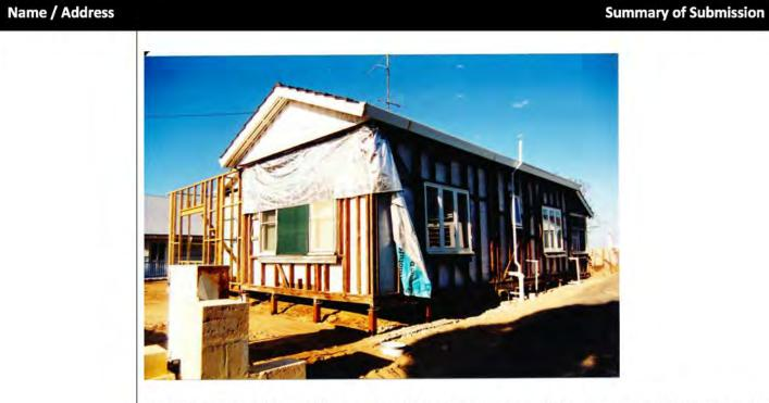
Photo 2: The condition of the property during a complete rebuild in the year 2000, removing the spalled brick work, installing new stumps, complete re-wiring, new windows, new wall insulation and new plumbing was installed.
