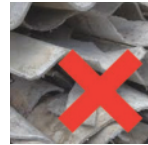
Asbestos and fence panels
