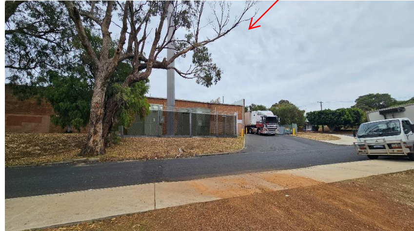
After – 35m structure
