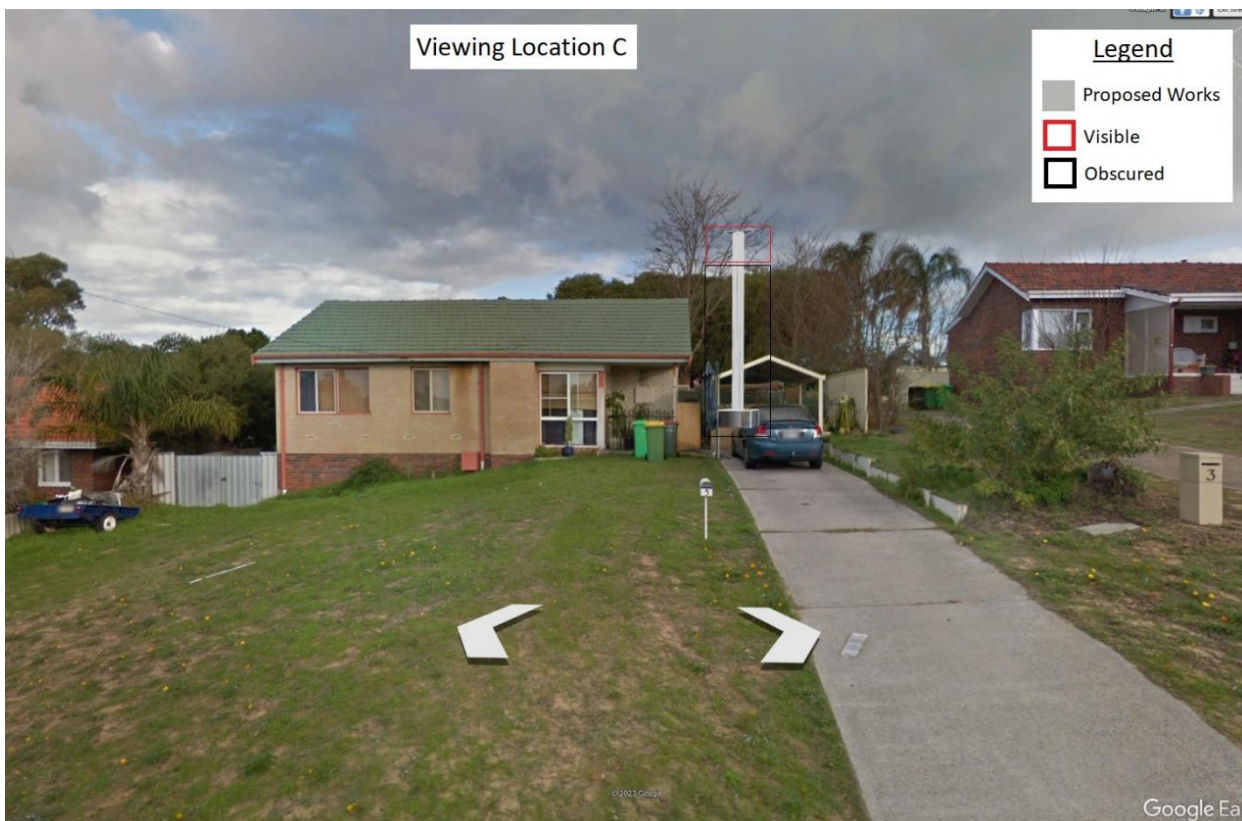
Figure 15: View looking South towards the proposal from Knight Street approximately 120m away - Source: Google Earth
