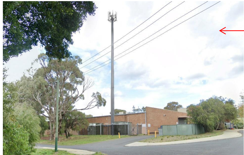
After – 35m structure
