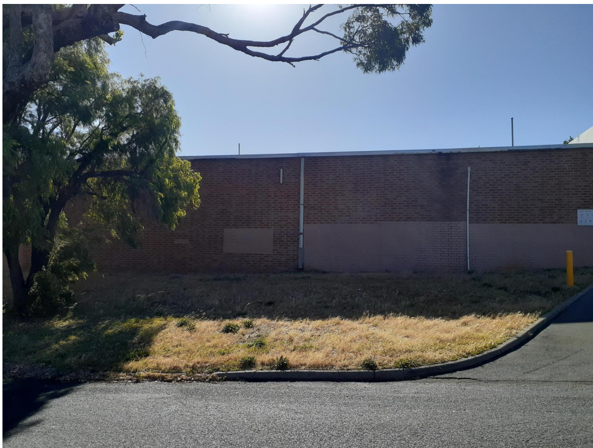
Devonshire Street Facing Proposed Location of Telecommunications Infrastructure
