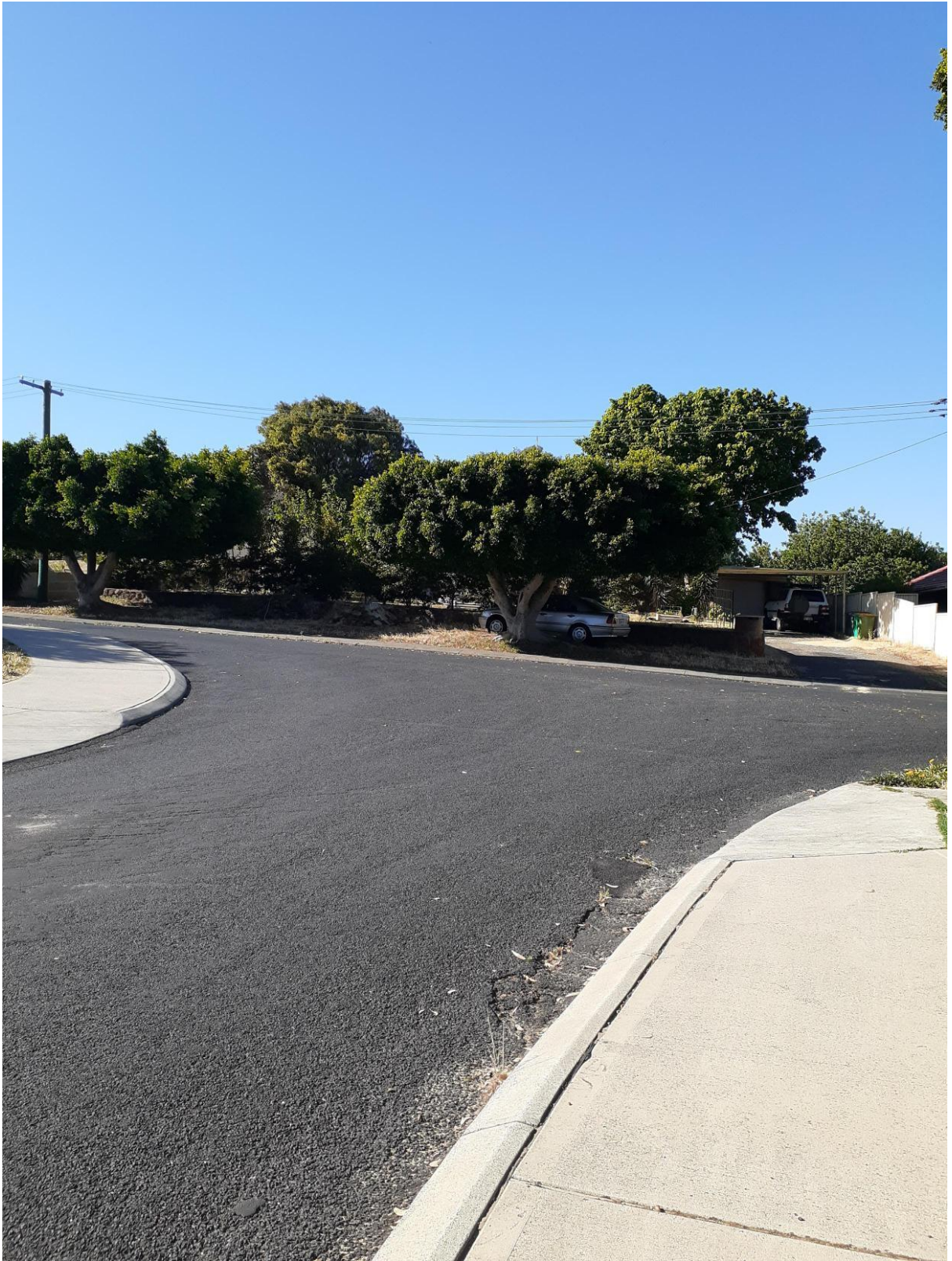
Intersection of Devonshire Street and Island Queen Street
