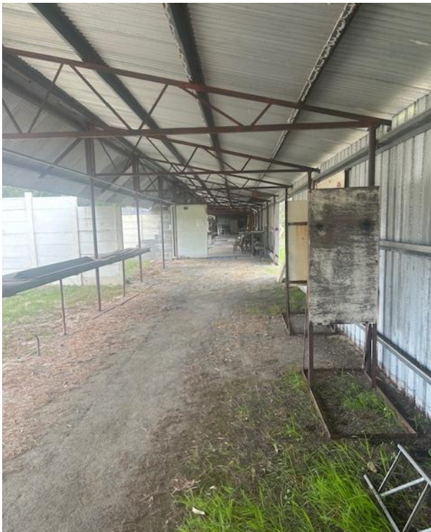
Figure 4 View down the full length of the shed
