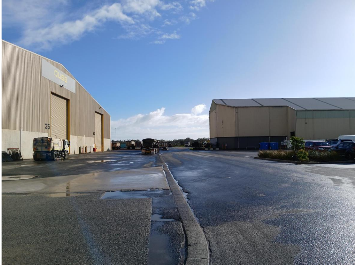
View of Rossiter Road facing North
