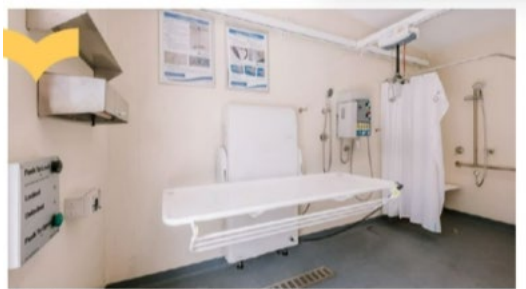
A Changing Places facility with an adult change table, ceiling hoist and shower.
