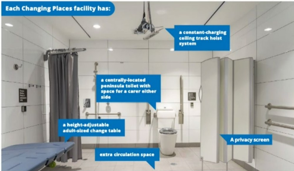
A typical Changing Places facility
