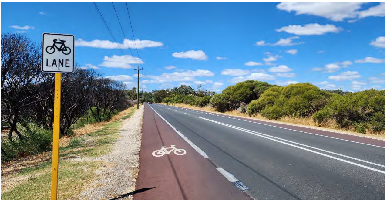
Photo 4: Washington Avenue, looking east.
