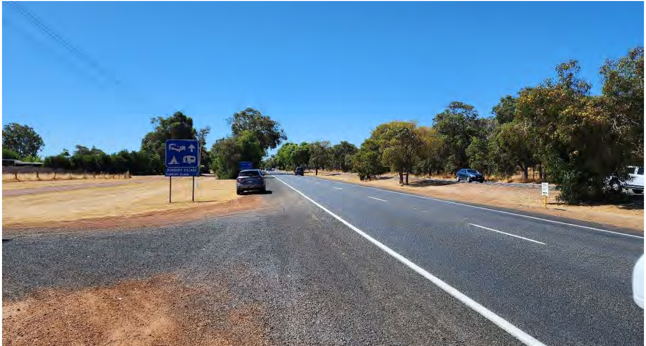
Photo 3: Bussell Highway northbound carriageway, looking north from a property access. Note PSP on left.
